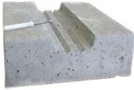
concrete footing + hammer plug
