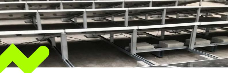
Align the rows according to plan, taking into account the width of the panels. To easily determine the distance between the basic units, you can use the Avasco Solar spacer.
